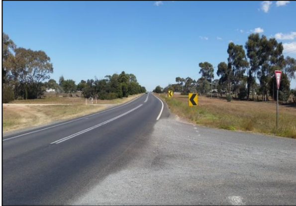
Figure 7: Geelong-Bacchus Marsh Road (near Smiths Road) – View South
