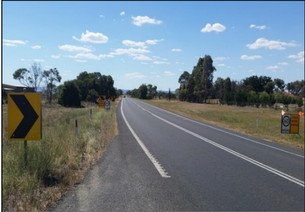
Figure 6: Geelong-Bacchus Marsh Road (near Smiths Road)– View North
