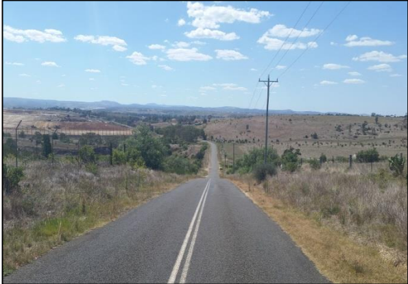
Figure 4: Cummings Road – View North
