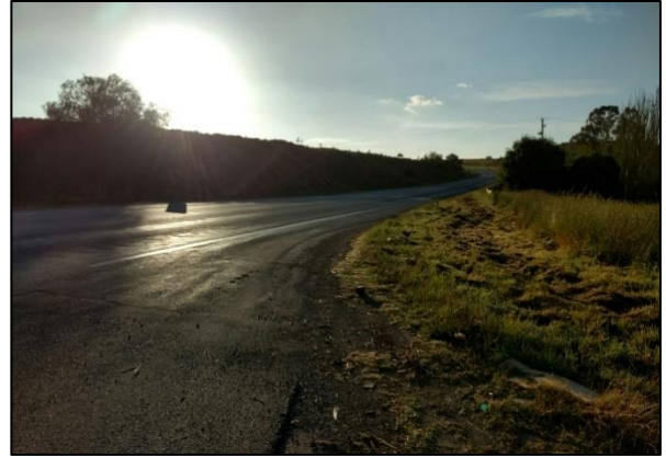
Figure 9: Geelong-Bacchus Marsh Road (near Cummings Road) – View East
