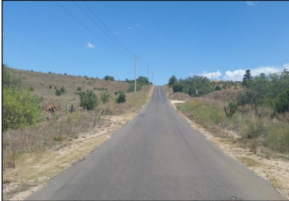
Figure 5: Cummings Road – View South
